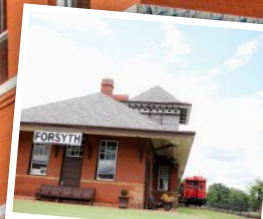
HISTORIC TRAIN DEPOT
